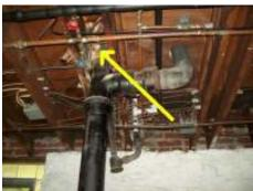
• The kitchen drain waste stack is leaking at the connections and needs to be repaired.
