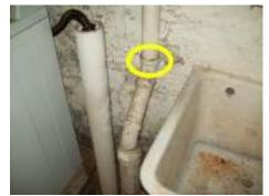
• The drain for the bathtub is sloped incorrectly and runs uphill. This may not allow the tub to drain properly. Repair is needed.
