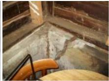
• There is damage from wood destroying insects on the rear wall framing of the garage. A portion of the damage has been reinforced.
