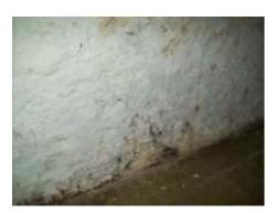
Moisture stains and efflorescence (The white calcium or mineral deposits that are left when water evaporates) were noted on the interior of the room under the front porch. The moisture is likely entering through the voids in the stone around the porch. The stone needs to be tuck pointed to discourage moisture from collecting in the openings.
