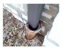
• The southwest downspouts do not appear to be tight to the underground drains which may allow moisture to bypass the drain and collect at the foundation walls. Recommend review of the underground drain and the connections to the downspouts.
