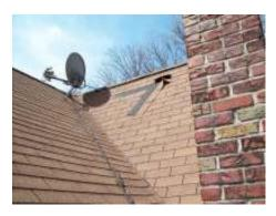
• The northeast plumbing vent is too short. The vent should extend a minimum of 6 inches to avoid being overtaken by snow.
