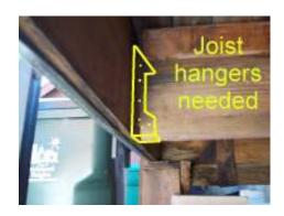
• The floor joists do not have a reinforced connection to the support columns. The floor structure appears to rest on shims placed in between the column without reinforcement. Brackets are recommended for the connections of the floor joists to the support columns.
