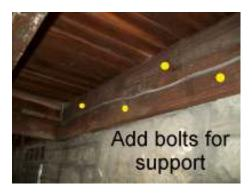
The deck was constructed without joist hangers to reinforce the connection of the floor joists to the ledger boards. Recommend adding joist hangers for added support.
