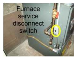
The condensate line for the flue pipe is leaking and needs to be repaired.
